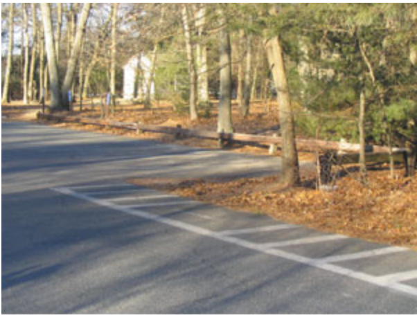
A look at a porous asphalt parking lot that is over 20 years old—Walden Pond (Concord, MA). Courtesy VHB.
