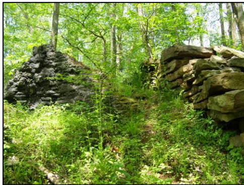
Remnants of Bassenheim Furnace, the first charcoal-fired blast furnace in western Pennsylvania
