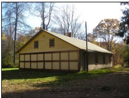
Civilian Conservation Corps structure in Croyland
