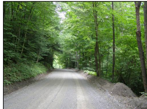
Proper management of the numerous dirt and gravel roads that are found throughout the region is important to control erosion and sedimentation
