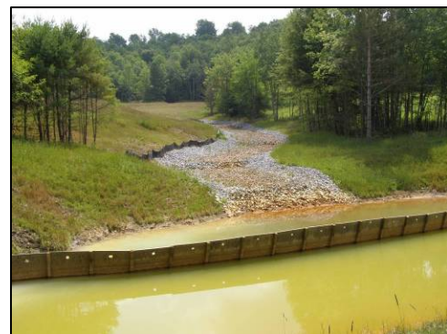
This settlement pond is one of many passive abandoned mine drainage treatment systems within the Bennett Branch subwatershed
