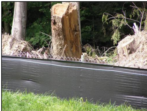
Siltation fences are used to control the loss of soil from a construction site. This particular siltation fence is termed a "super siltation fence" and is located at an AMD remediation project within the Bennett Branch subwatershed
