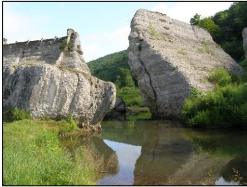
Remnants of the Austin Dam
