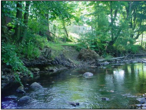
Streambank erosion along Dents Run
