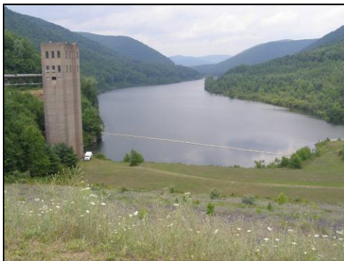
George B. Stevenson Dam at Sinnemahoning State Park on First Fork Sinnemahoning Creek
