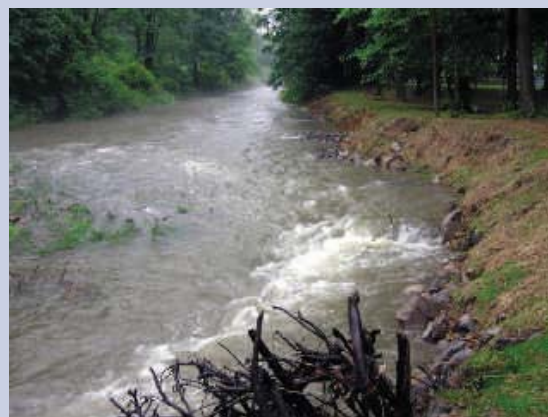
Before, during and after — WPC stabilizes a streambank along Mill Creek.
