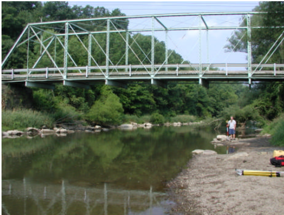
Figure 5. Photograph of French Creek channel at cross section location #1. View is looking downstream (west).
