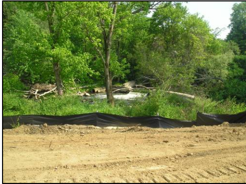
Silt fence to control sediment entering stream near a construction site
