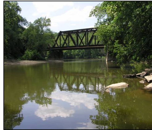
Connoquenessing Creek drains into the Beaver River just beyond the railroad bridge
