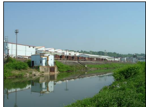
AK Steel Corporation Butler Works
