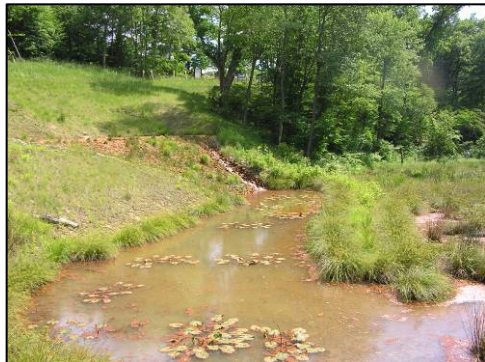
Passive AMD treatment system at Lutherlyn
