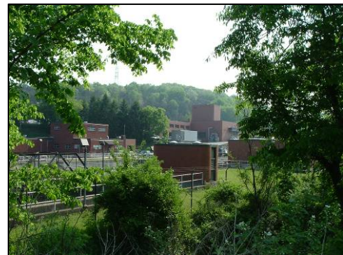
Butler Area Sewage Treatment Plant
