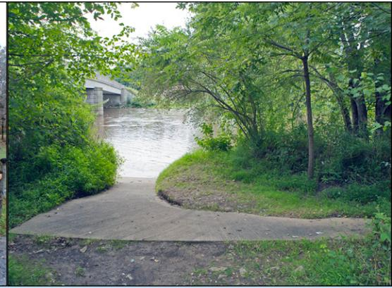
*The concrete at this access site in Utica, Pa., has striations to help prevent slipping when entering and exiting the water.*
