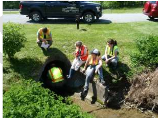
Photo 5-2. NAACC assessments determine if road/stream crossings pose a barrier to AOP.
