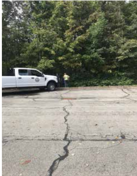
Catch Basin in the Center of Cedar Grove Lot, just above the Outfall Pipe
