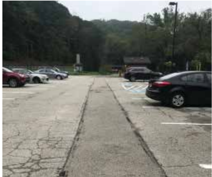
Chestnut Grove Parking Lot, slated for 2022 upgrades.
