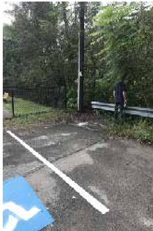
Parking Lot Catch Basin
