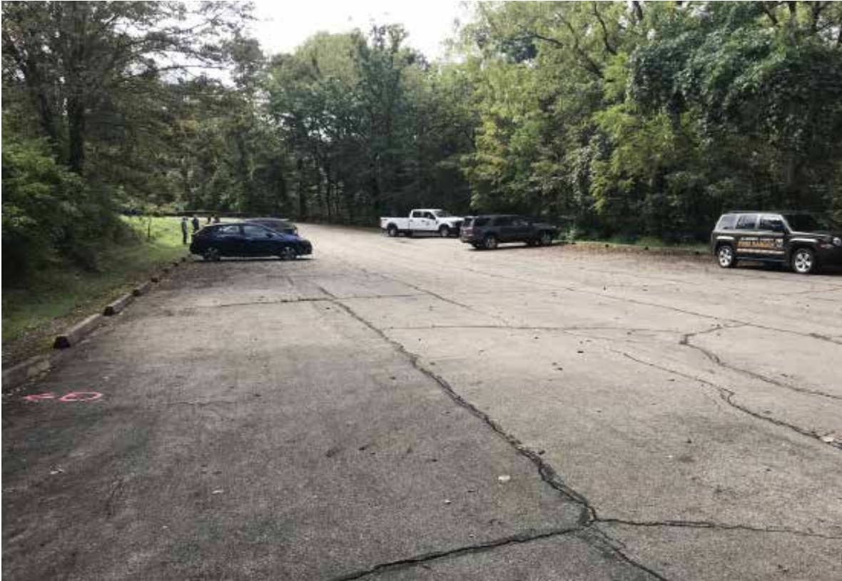
Cedar One Shelter Parking Lot
