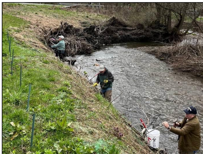
Volunteers transplanting live stakes of riparian shrubs to control erosion on Trout Run (photo: WPC)
