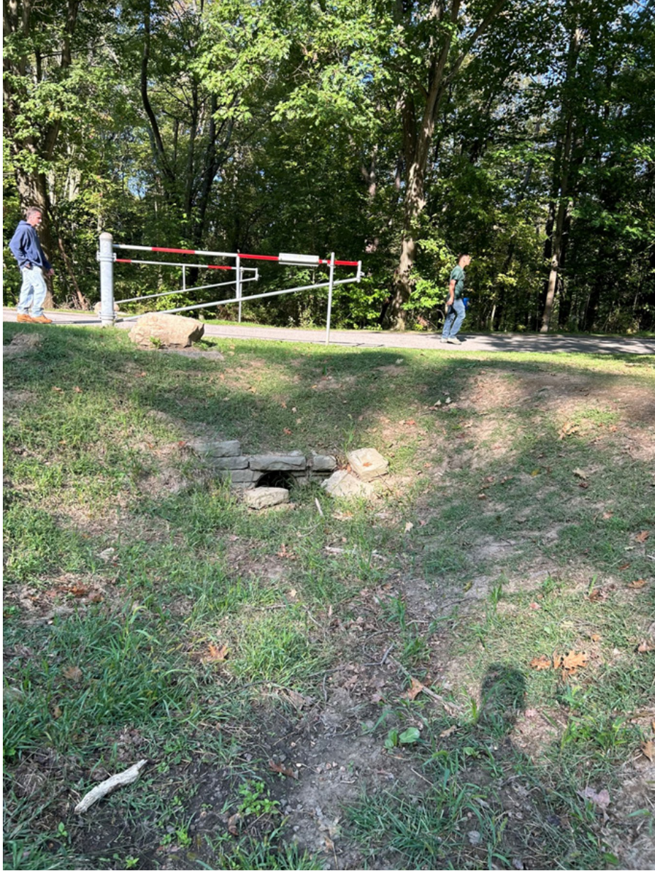
Erosion at the culvert under Crayfish Drive, with the wooded area beyond.
