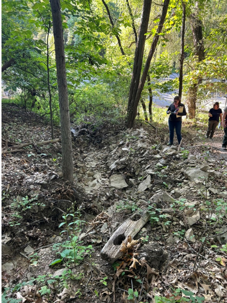
Substantial erosion on the slope between the Blue Gill Shelter and the parking lot. Check dams would slow and retain any runoff not managed by the introduction of the rain garden, berm, and retentive grading above.
