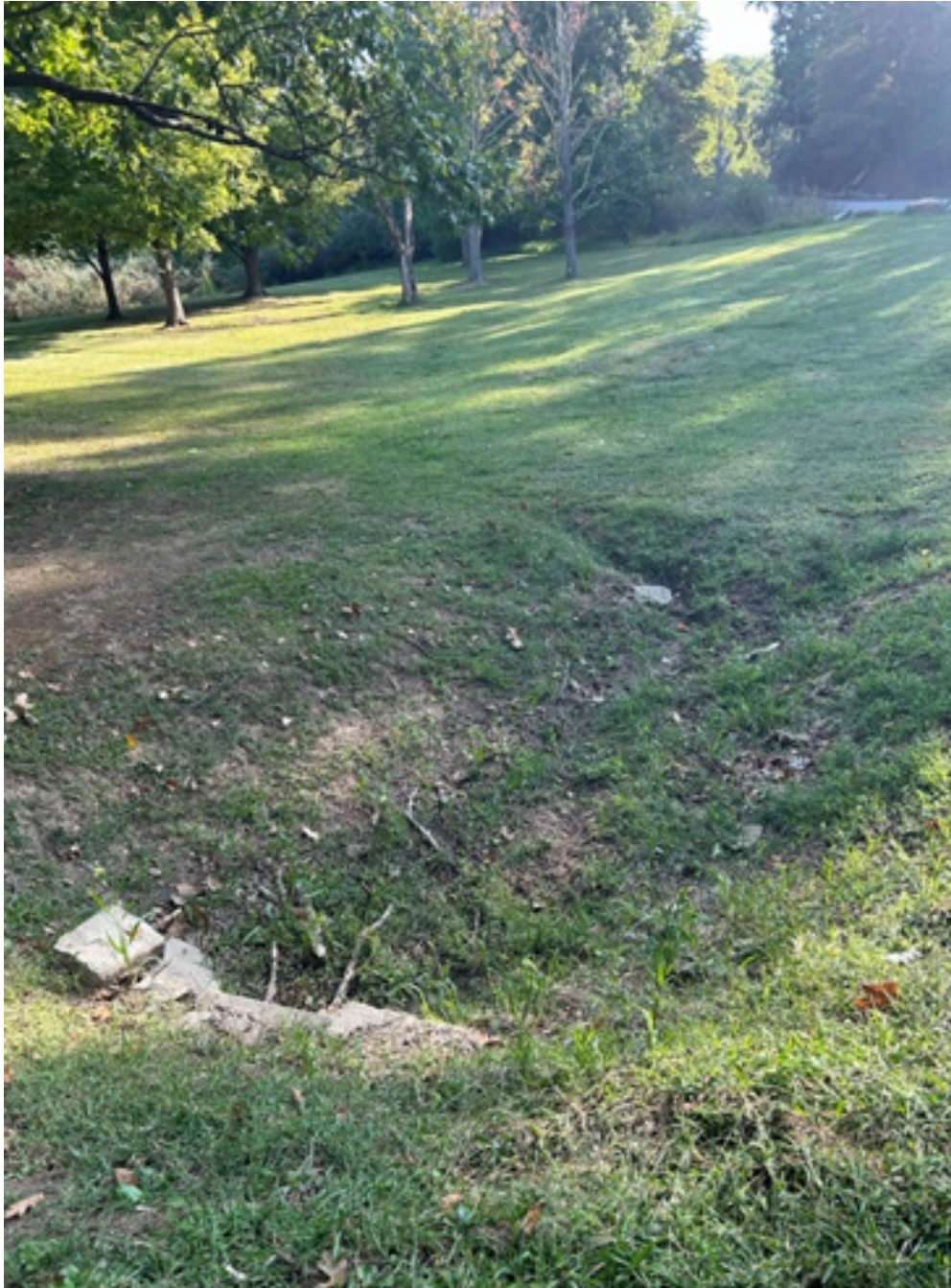
Erosion present at the culvert going under Crayfish Drive. Kurn Road is in the upper right corner of the photo.
