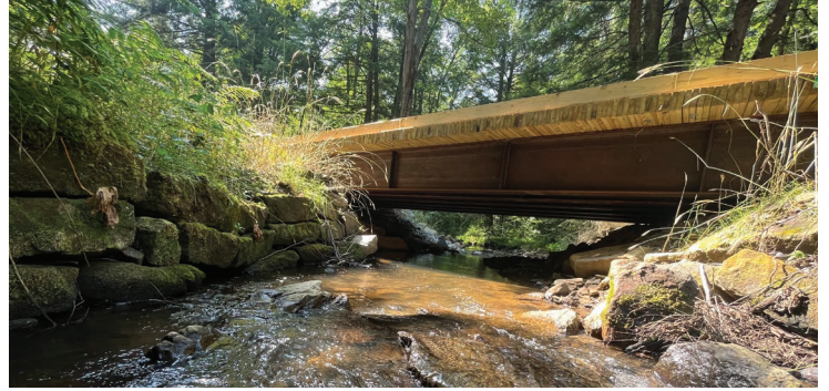
One of the bridges WPC and partners built to replace deficient culverts on the Middle Fork East Branch Clarion River on State Game Lands 25, reconnecting 12 miles of stream.
