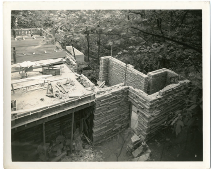
This historic photo from the original construction reveals the rubble in the walls, soon to be injected with grout.
