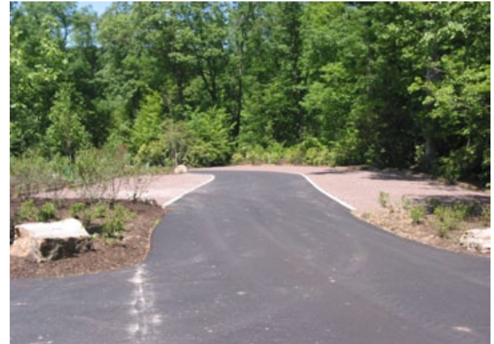
Permeable parking spots at Fallingwater. Photo: WPC.
