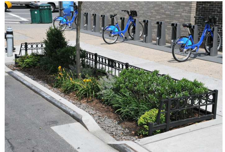
Example of stormwater inlets on a tree pit at Atlantic Avenue and Dean Street. Photo: NYC Water.
