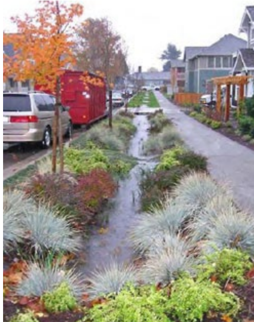
Examples of vegetated bioswales. Iowa Association of Municipalities (left), and Nebraska State-wide Arboretum (right).
