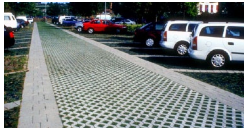
Example of open cell porous paving. Photo: Unknown.
