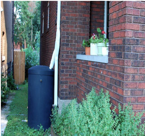
Rain barrel collecting water from a disconnected downspout as a community effort to divert rain water in the Nine Mile Run watershed. Photo: Katy Frey.
