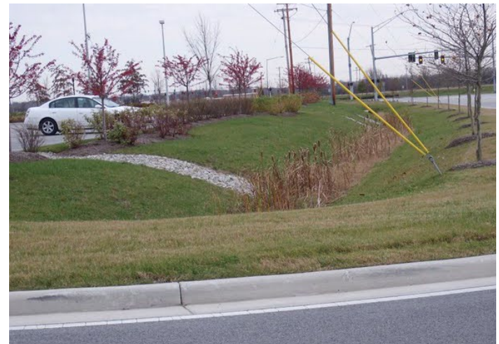
Bioswale example between a parking lot and street. Photo: Jennifer English, Defiance (OH), Storm Water Conservation District.
