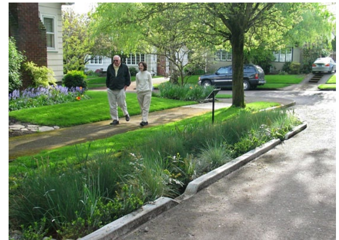
Street bumpouts with stormwater inlets in Portland, OR. Photo: Kevin Robert Perry.
