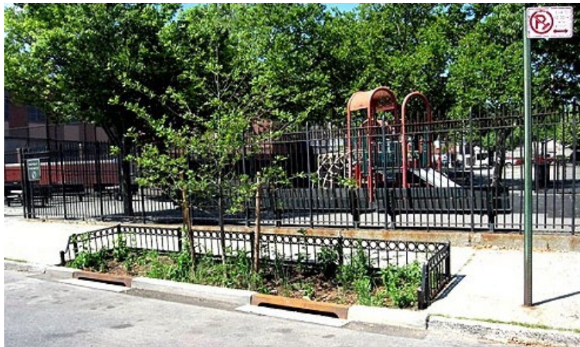
Stormwater tree pits with inlets at Autumn and Stanley Avenues, East New York, Brooklyn. Photo: City of New York.
