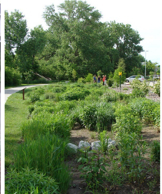
Examples of vegetated bioswales. Iowa Association of Municipalities (left), and Nebraska State-wide Arboretum (right).
