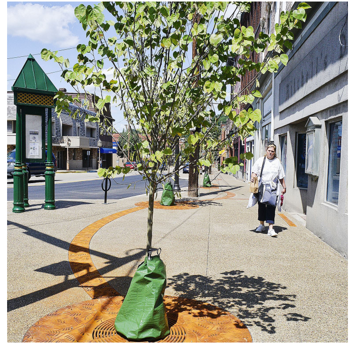
New stormwater capture grates in Etna. Photo: Larry Roberts, Post-Gazette.
