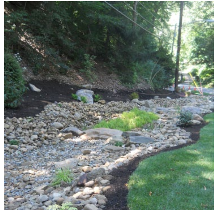
400-foot long bioswale along Hawthorne Drive in Millvale. Photo: WPC
