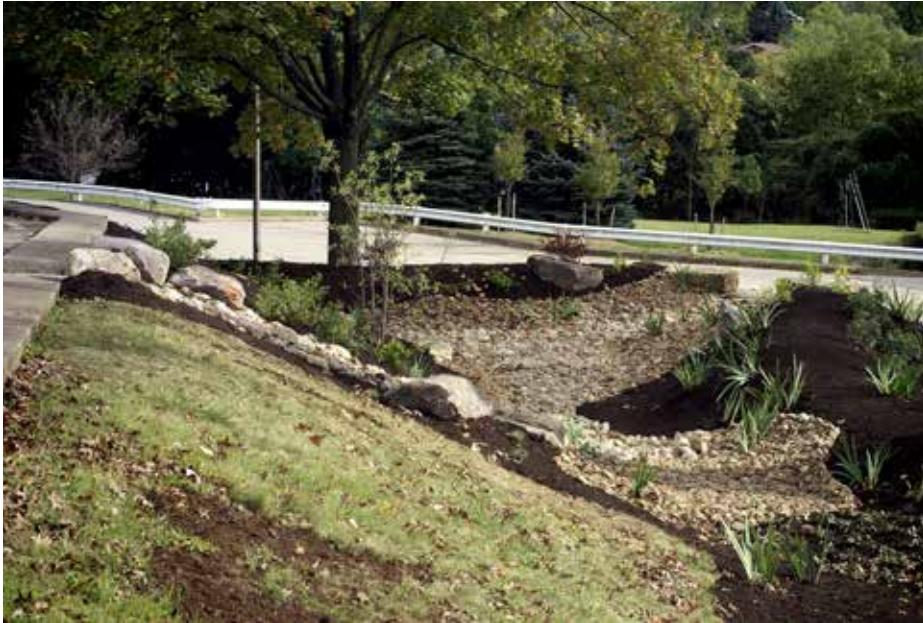
Bioswale installed by WPC on the edge of a parking lot in Millvale. Photo: Matthew Little.
