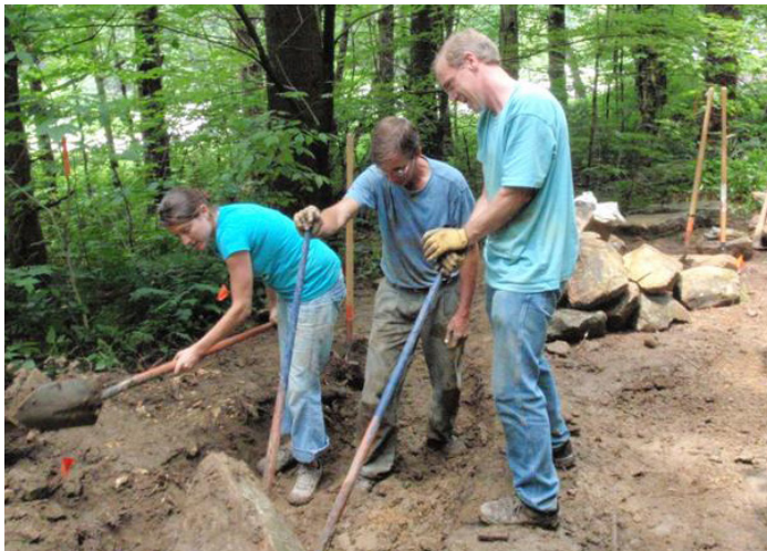
Volunteers Chelsea Attwood, Bob Chesky and Dan Nydick install open stone culverts at Bear Run Nature Reserve.
