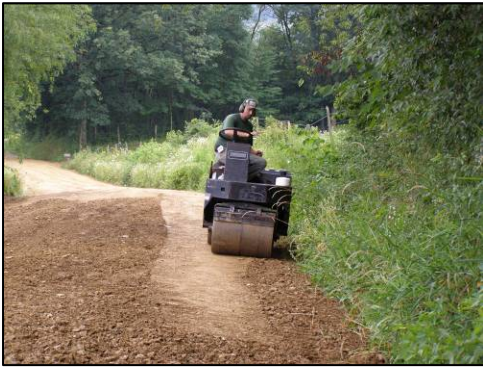
Mottarn road dirt and gravel road project during construction phase in July 2008, where 11 culverts were installed and the roadway was re-graded
