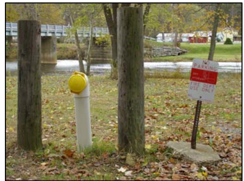
Dry hydrant located at Putneyville Park is used by firemen needing access to water in emergency situations where there is no public water system and a lack of fire hydrants
