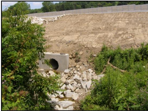
Highway construction can have direct sediment impacts to streams when proper erosion and sediment plans are not followed.
