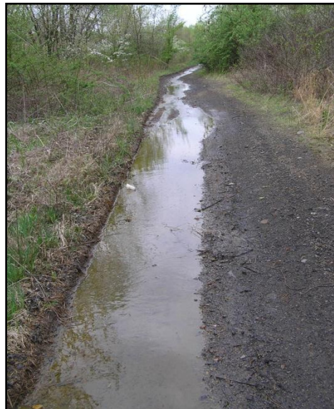
A headwater tributary of the North Fork of Sewickley has eroded its bank and travels along a paralleling mining site access road for several hundred feet before entering back into its original channel.
