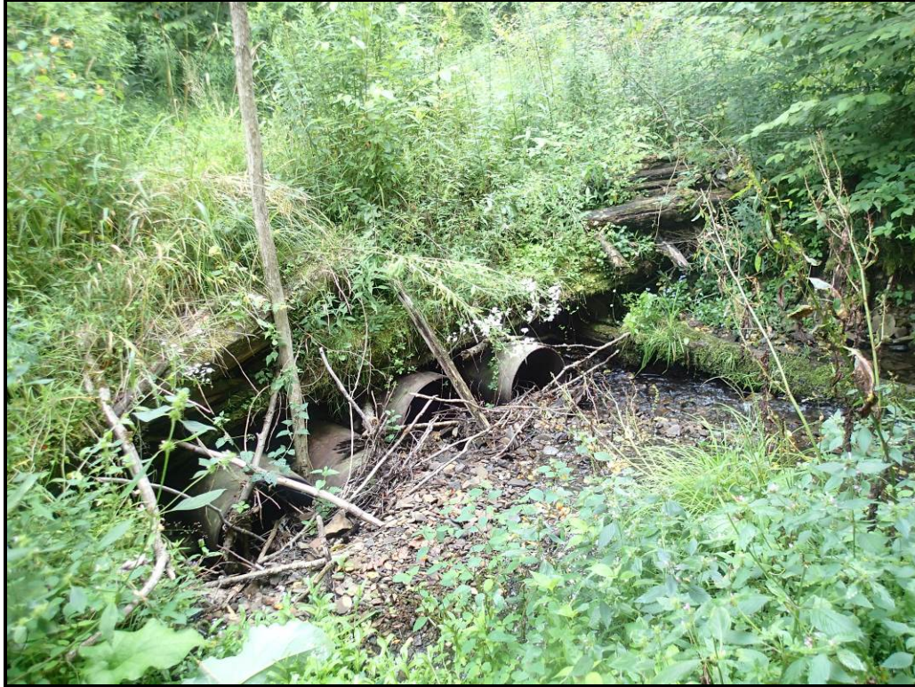
Figure 23. Debris choked culvert on Little Parker Run
