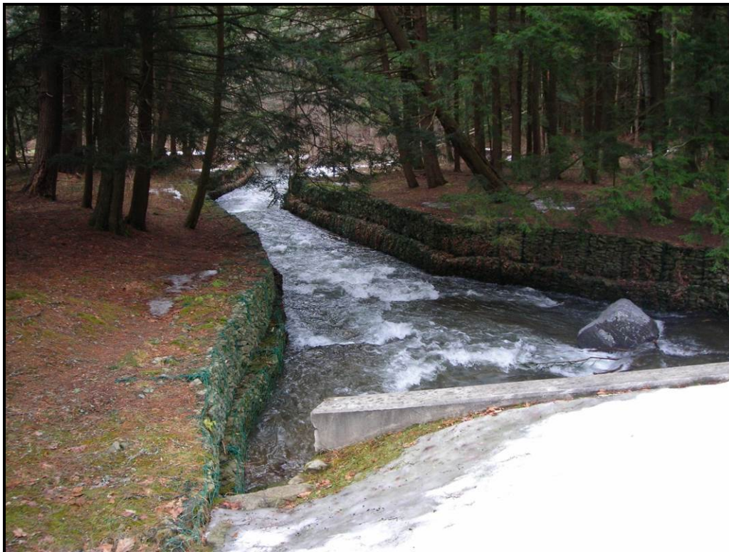
Figure 37. Streambank stabilization using gabion baskets in Sizerville State Park, segment 1090
