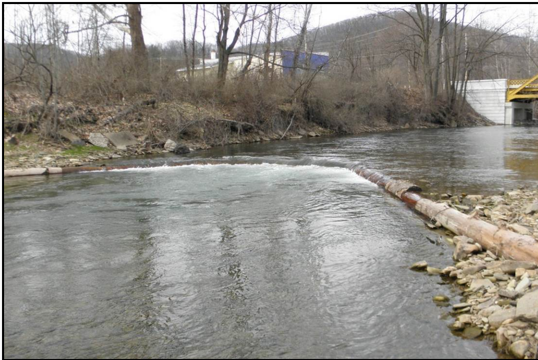
Figure 70. Log cross vane project completed by Cameron County Conservation District on segment 1526
