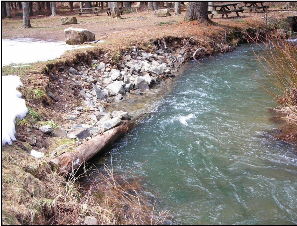
Figure 38. Severe bank stability issues evident with this failed mudsill along stream segment 1090
