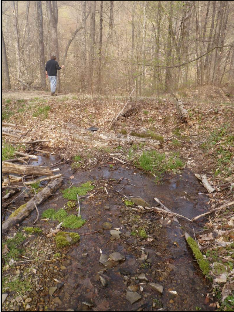
Figure 21. Debris choked culvert on segment 1149
