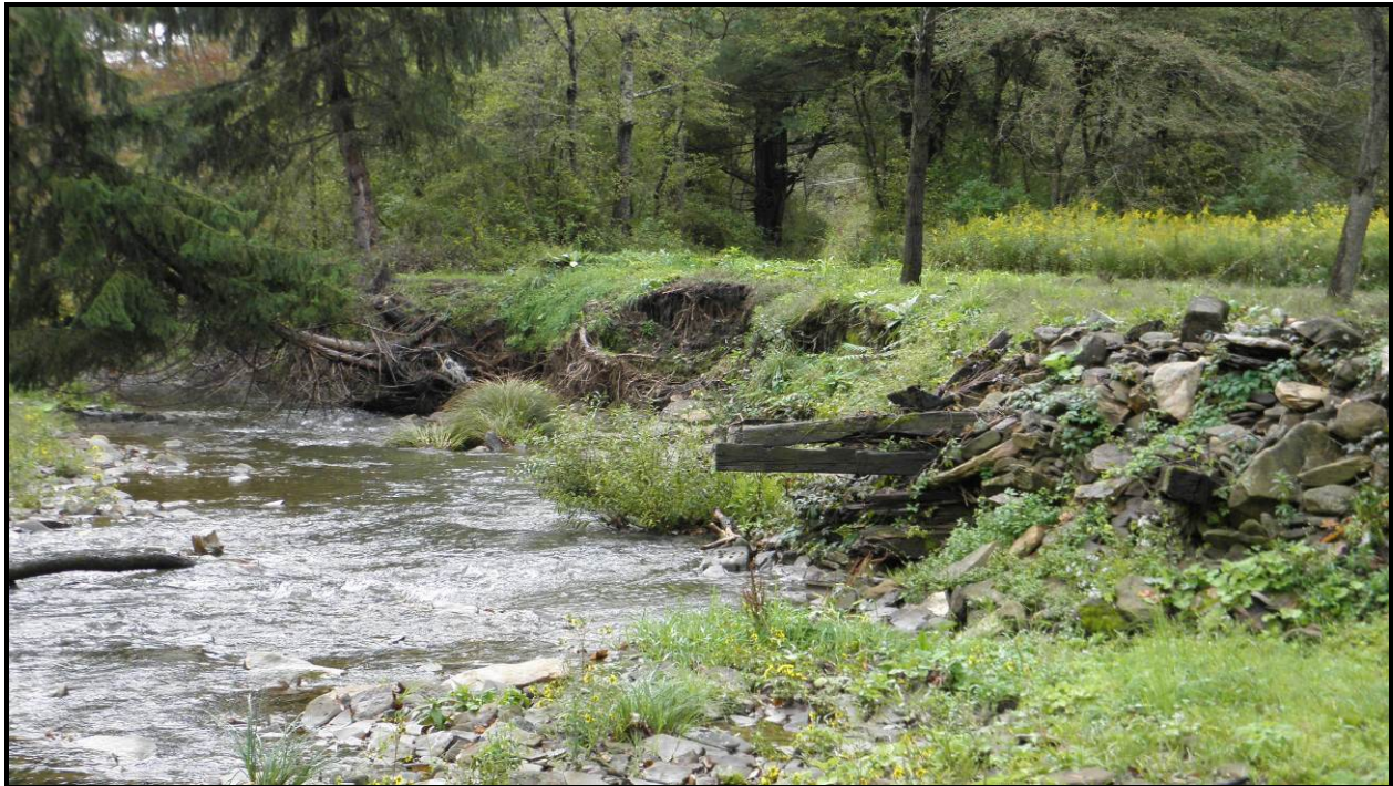
Figure 65. Streambank erosion and failed stabilization efforts on segment 1693
