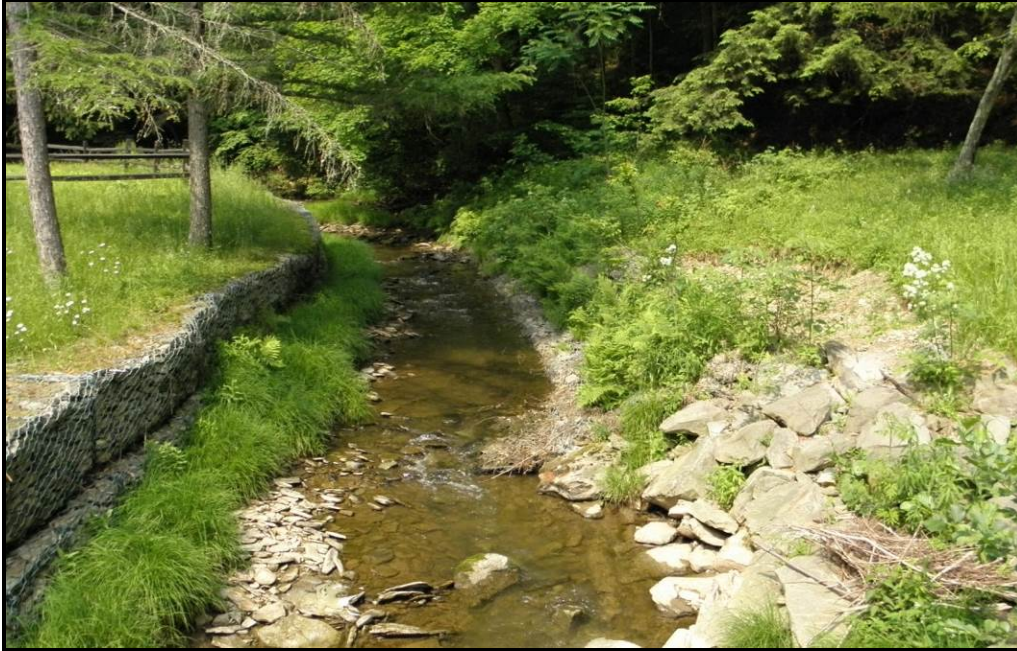
Figure 31. Gabion baskets and riprap serve as bank stabilization on segment 1002
