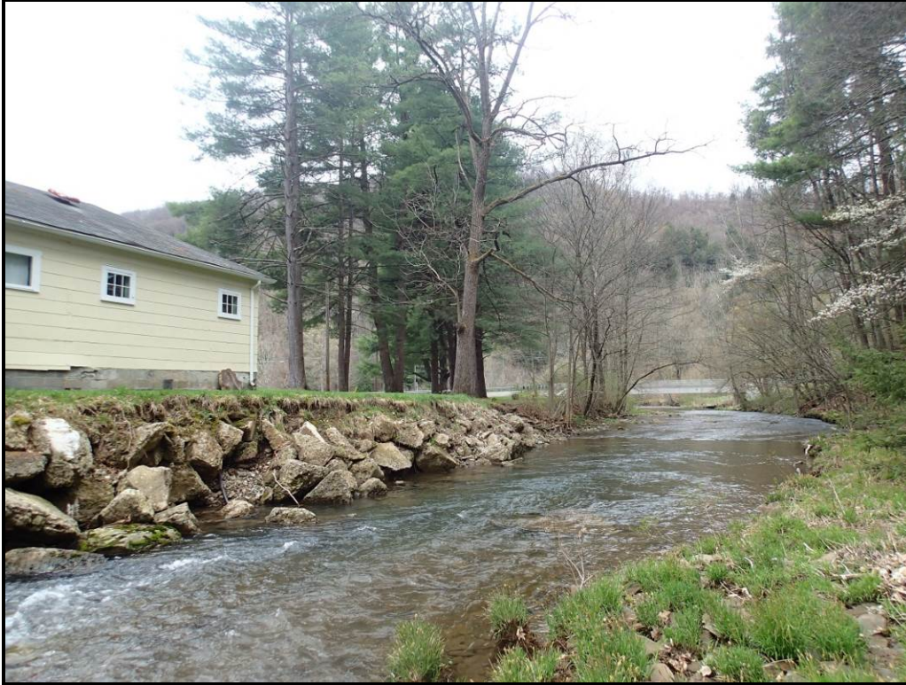
Figure 27. Rip-rap stabilization and riparian zone encroachment on Cowley Run, segment 1708
